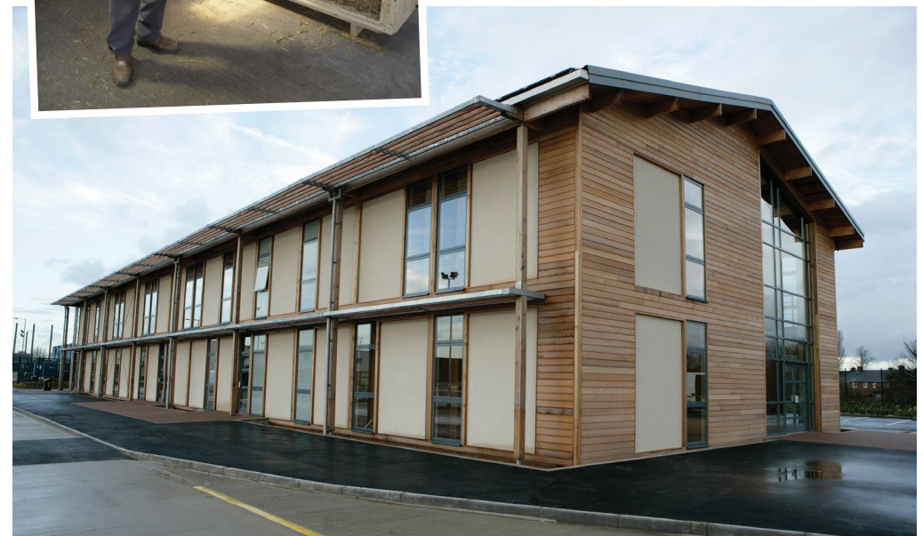
York City Council's Eco-depot, one of Europe's largest timber frame straw bale clad buildings.
